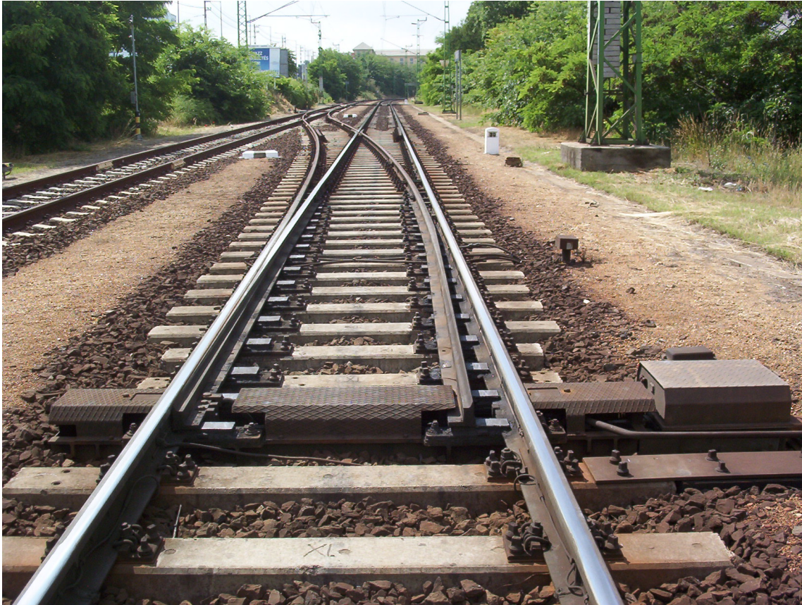
Figure 1.1. A junction's facing-point with blades pointing to left – the straight way – at Budapest-Soroksári út railway station
