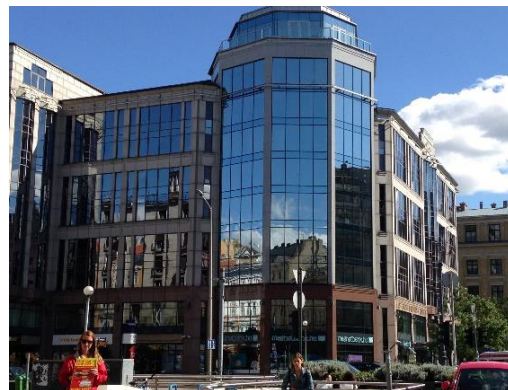
8. ábra: Zalaváry Lajos- East-West Business Center
