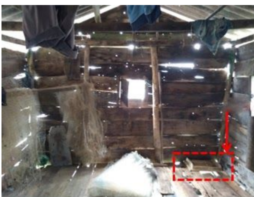
Picture 1-04 Toilet disposition Buenavista. 25
