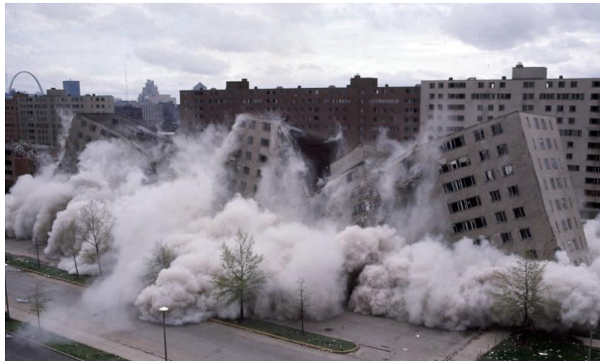
Figure 3.8. The Pruitt-Igoe housing project in St Louis, Missouri, being demolished with explosives. Photograph: Lee Balterman/The Life Images Collection/Getty.
