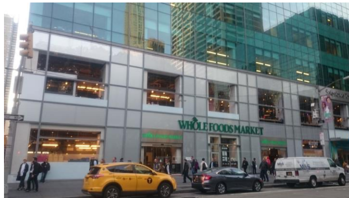
Figure 3.20. Whole Foods Market building, New York; [20]
