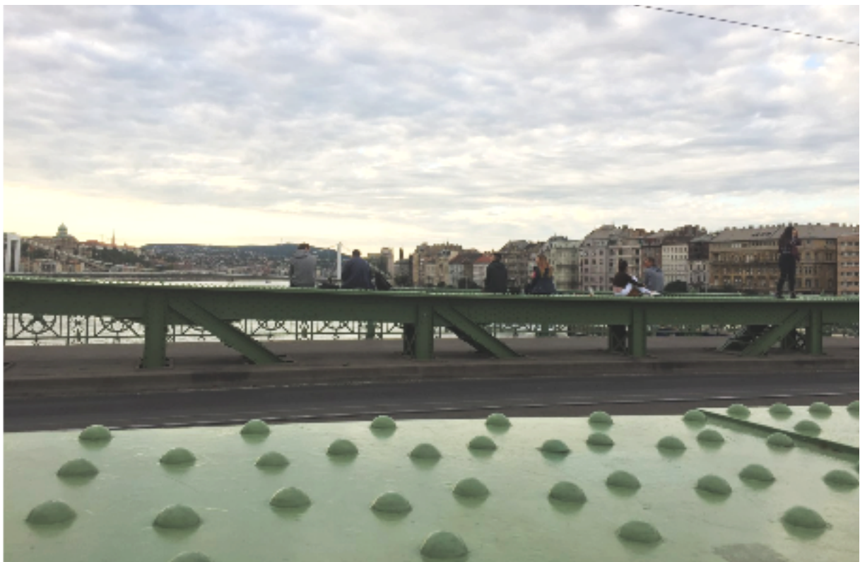
Using Liberty bridge as a seating surface, source: author's own photo
