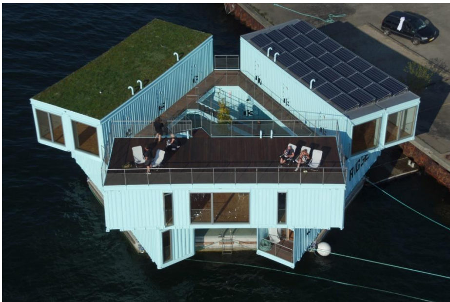
Jessica Maris: BIG stacks containers to create floating student housing in Copenhagen harbour; 2016.09.22., Dezeen ( https://www.dezeen.com/2016/09/22/big-bjarke-ingels-shipping-containers-floating-student-housing-urban-rigger-copenhagen/ ) (letöltés időpontja: 2020.10.25.)
