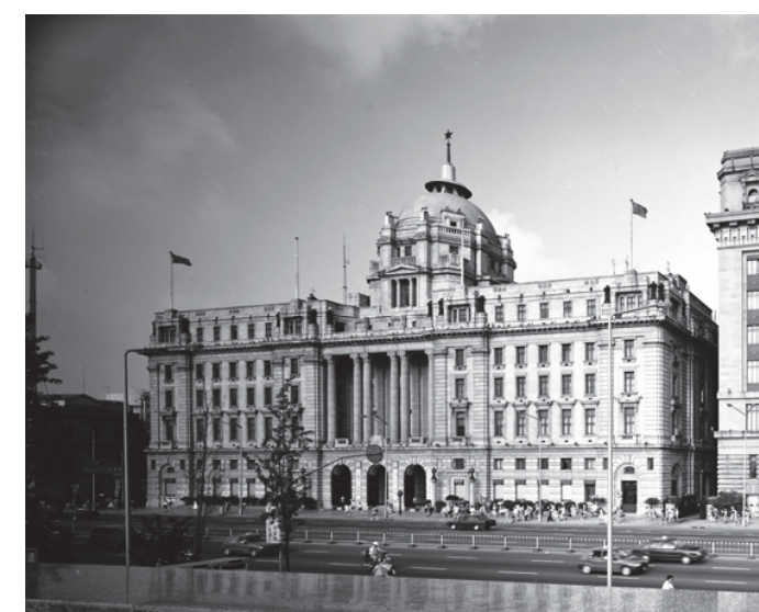
32.picture – 32.kép The façade of the HSCB by P&T A HSCB homlokzata, P&T
