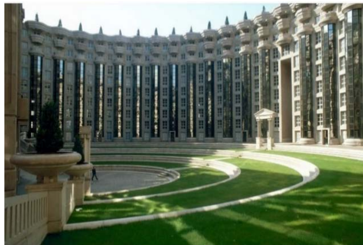
Figure 5.5. Residential complex "Theater" (Marne la Vallee, architect Ricardo Bofilla). [25]
