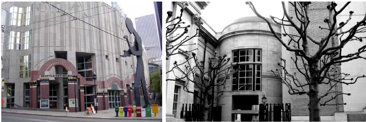
Figure 5.3. From left to right: Seattle Art Museum (Washington, 1991) [19]; Sainsbury Wing (London, 1987-1991). Architects: R. Venturi, D. Scott-Brown. [20]
