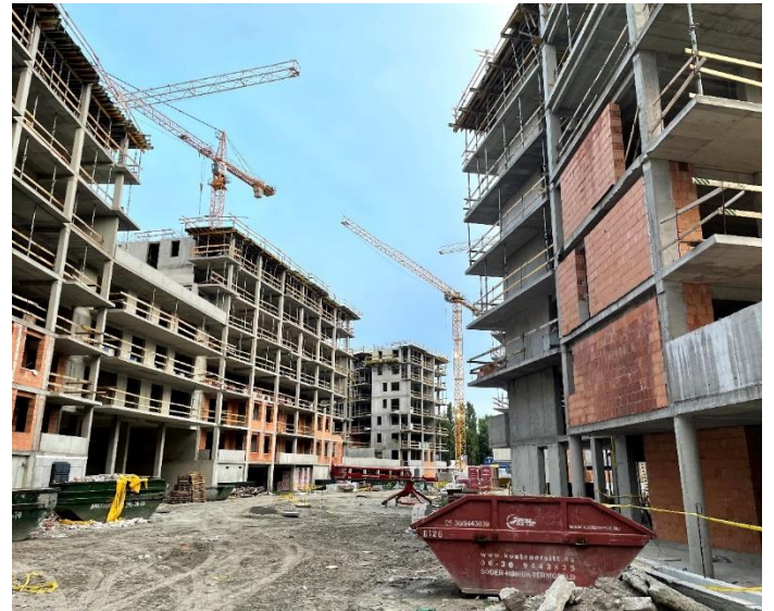
Figure 13 : 8 storey buildings under construction with roof gardens connected between them . Source: The Author (August 2021)
