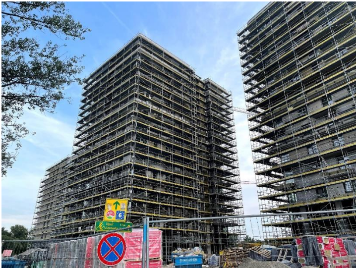
Figure 10 : Waterfront City project under construction Source: The Author (August 2021)
