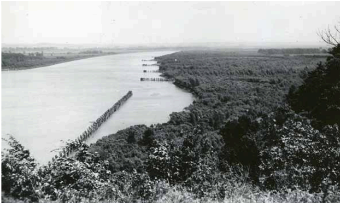
Fig. 49 (A-D).: The siltation of a dike system, Indian Cave Bend, Missouri River. [15]
