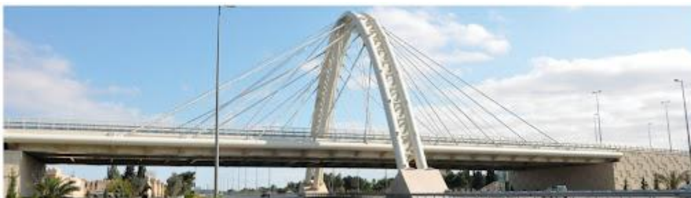
9. ábra: Bine Bridge [12]
