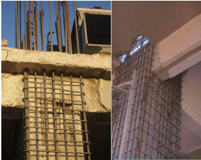
Figure 2-1: Total jacketing of concrete columns in practice (Dritsos, 2015)
